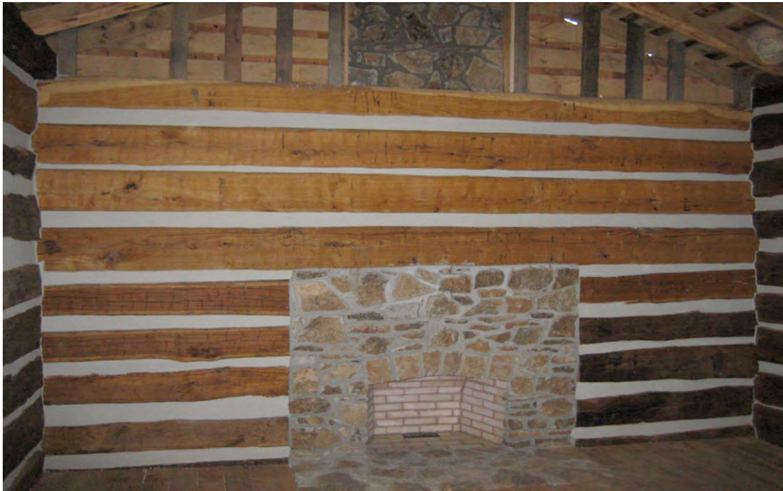
Inside East Wall with fireplace.
